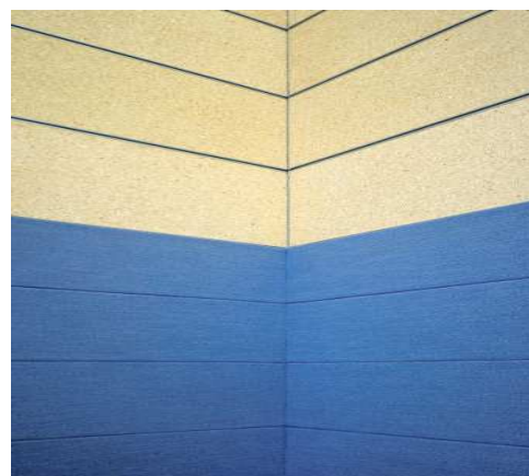
Sporthalle Uckermark Kaserne Prenzlau Detail Innenecke
